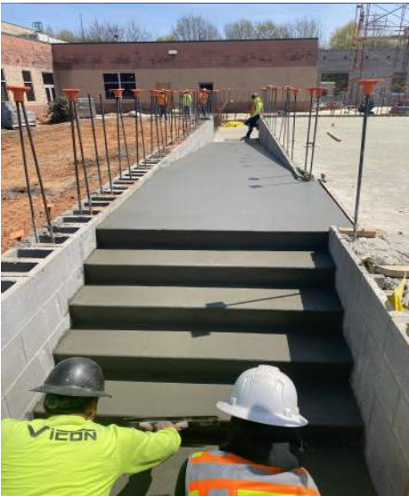
Gym stage ramp and stairs poured
