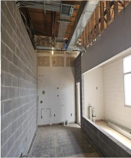
Drywall installed in the serving line area
