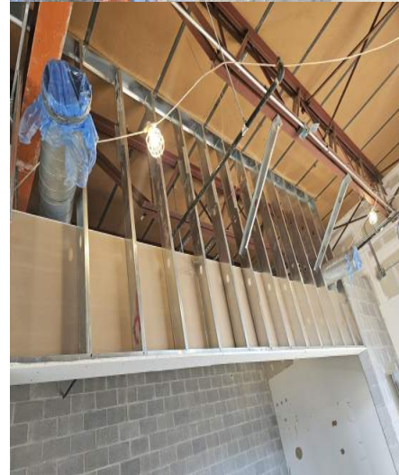
Metal framing installed in serving line area
