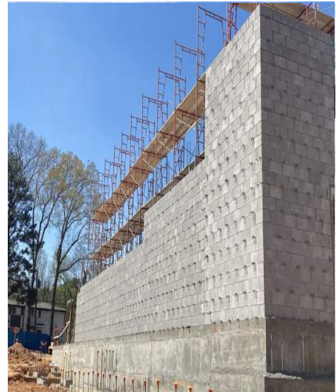
CMU Exterior Walls being installed
